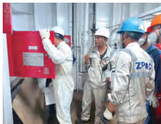
The commissioning team is conducting carbon dioxide inspection in the engine room
